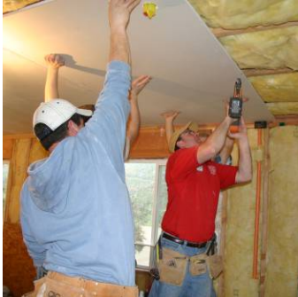
(Mennonite Disaster Service photo)
