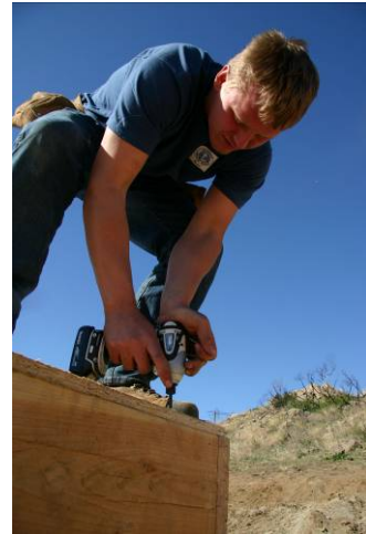
(Mennonite Disaster Service photo)
